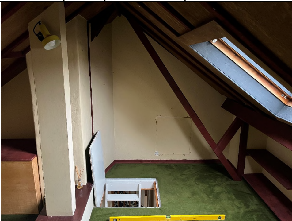
Figure 2 – Floored semi-finished loft, access hatch and fixed ladder.
