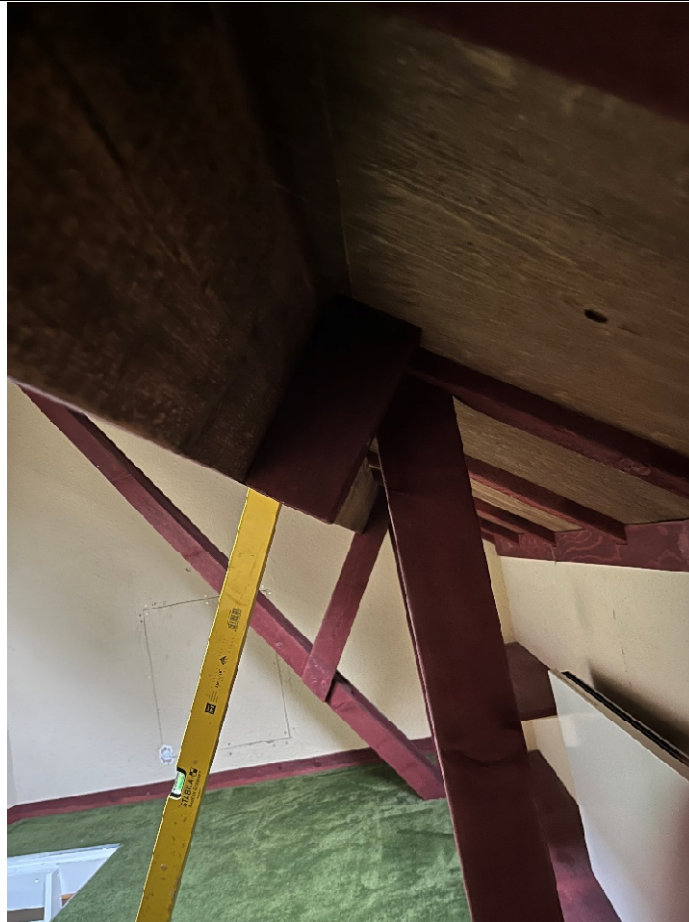
Figure 3 – Evidence of removed internal roof members.
