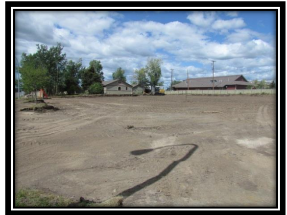
LOOKING TOWARDS NORTHWEST CORNER
