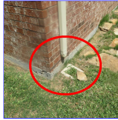
B. Item 3 (Picture) Missing sections, extensions & pads reversed
