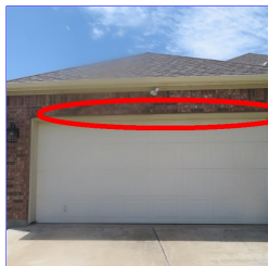
G. Item 1 (Picture) Tops of lintels at doors not sealed
