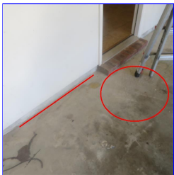
F. Item 2 (Picture) Hairline cracks
