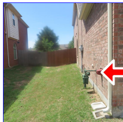
E. Item 1 (Picture) Meter not bonded
