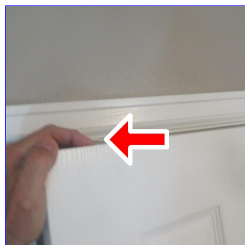
G. Item 4 (Picture) Missing/damaged ball pressure latches
