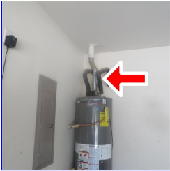
C. Item 1 (Picture) Not type B flue in garage & no sediment trap on gas line
