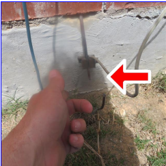
A. Item 1 (Picture) Grounding wire has been cut
