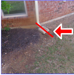
B. Item 1 (Picture) Missing extensions & pads reversed
