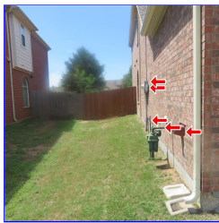
E. Item 4 (Picture) Seal all fixtures at exterior walls
