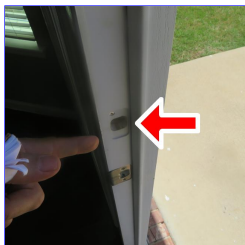
G. Item 2 (Picture) Sticking back door missing hardware
