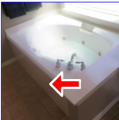
D. Item 1 (Picture) No visible access panel & slow draining
