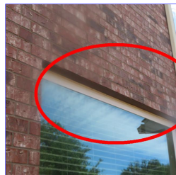
H. Item 1 (Picture) Tops of lintels at windows not sealed
