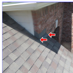
C. Item 1 (Picture) Missing kickout flashing
