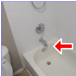
A. Item 5 (Picture) Leaking diverters
