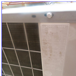
B. Item 2 (Picture) OLD 2005, rusting & bruised AC using R-22 freon
